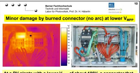
At a PV plants with a lower  $V_{MPP}$  of about 100V, a connector that joins the two halfs of the array in the middle of the connector box burned and caused an interruption (see thermographic picture at left, repaired connector box with wires replacing the defective connectors at right). Due to the lower  $V_{MPP}$ , no arc and no fire has occurred in this case.
