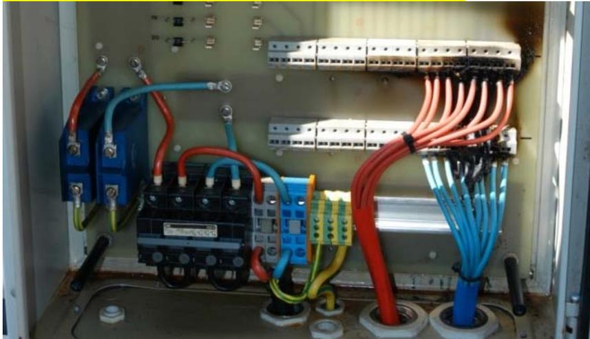
Damage caused by a smouldering fire, which occurred in the connector box of an 11 year old PV plant (15kW) in Burgdorf.
