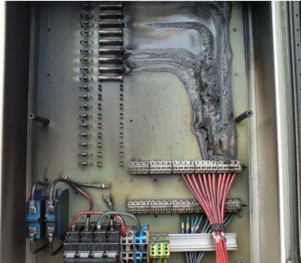
**PCB tracks already charred by series arcs in an array connector box of a similar PV plant of 20kW ( $V_{MPP}$  about 500V) immediately after opening of the cabinet. In this condition, the PV power was already very much reduced.**
