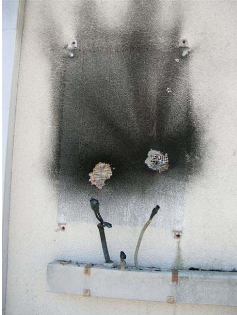
**Damage at the outer wall (with external thermal insulation) of the building, on which the connector box was mounted. The arc in the cabinet even melted a hole through the back wall of the metal cabinet!**
