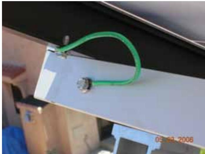
*Figure 4:* Connection of dissimilar (incompatible) materials, before corrosion begins.
