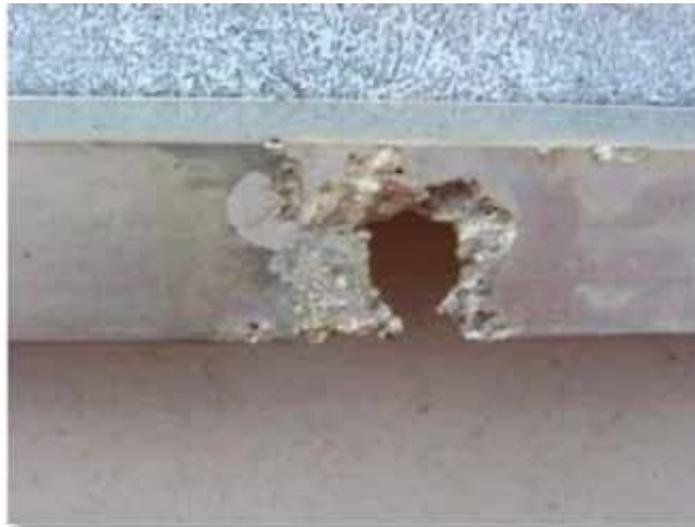
*Figure 3:* Lost connection from corrosive bond.
