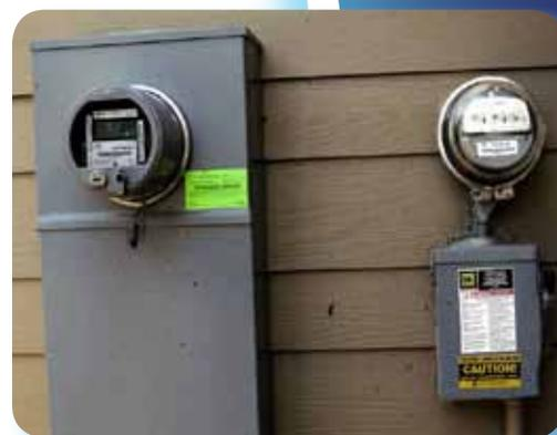
*Figure 1: Typical location of Utility External Disconnect Switch, marked with a yellow caution label, below the production meter. The revenue meter is to left.*
